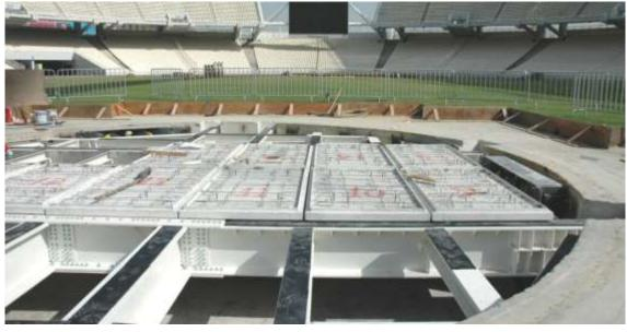
Concrete chamber for the opening ceremony of the Olympic games in the center of the stadium field. There can be discerned the elevator guides and the steel structure for the coverage of the chamber's roof
